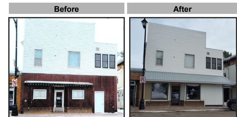
(Below) MRC Prop LLC (Barron County) — MRC Prop LLC is solely owned by JoDee Peterson-Lochner. The business owns a commercial building in downtown Turtle Lake. A Façade Loan assisted with a new store front inclusive of windows, doors, awning, and siding. In-progress renovations are pictured below.
